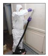
Paint sealant around the hole before you insert the screw. Use shadow vacuuming (if Class H vacuum available) to control dust when removing screws
