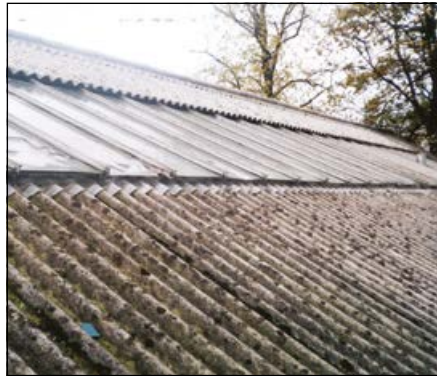
AC sheets used as roofing
