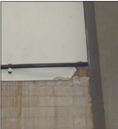
This damaged AIB needs to be covered and protected from further damage
