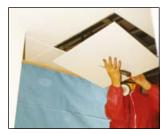
Carefully lower one end of the tile. Vacuum its upper surface and spray with PVA. Keep the tile flat and lower it gently
