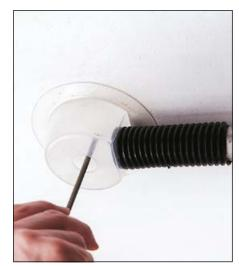
Protect nearby areas with polythene sheeting or a mini-enclosure. Use shadow vacuuming to control dust when removing screws
